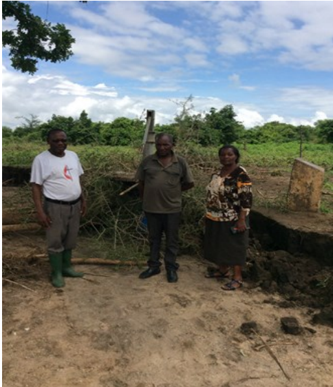
Umba, Msasa (well construction engineer), and Pastor Idda, standing in front of the well that was destroyed. Through your generous support, we are in the process of repairing it.
